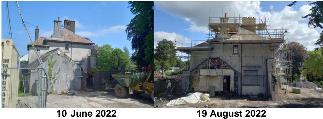
Fig. 3 – Photographs of western gable end of Listed Building
